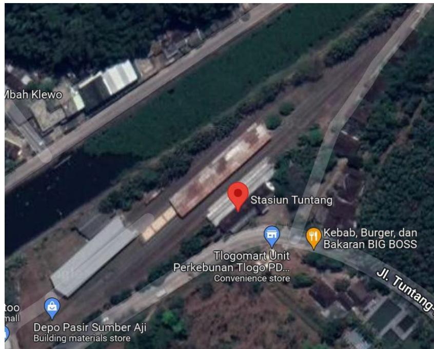
Tuntang Station (Source: Google Maps)
